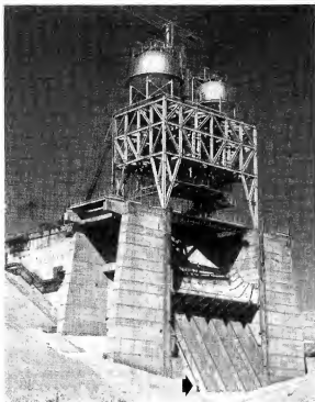
The F-1 test stand in the Mohave Desert towered 76 meters (note man at base).
